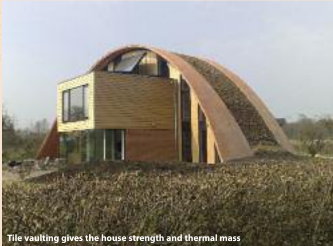
Tile vaulting gives the house strength and thermal mass
